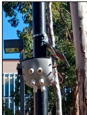
Figure 8. Proposed system installed on the electric pole.
