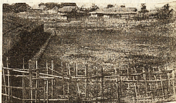
Fig. 8.—The southernmost arm of the bhil below the bazar cooly lines: a contour-drain protects it, as seen on the left.
