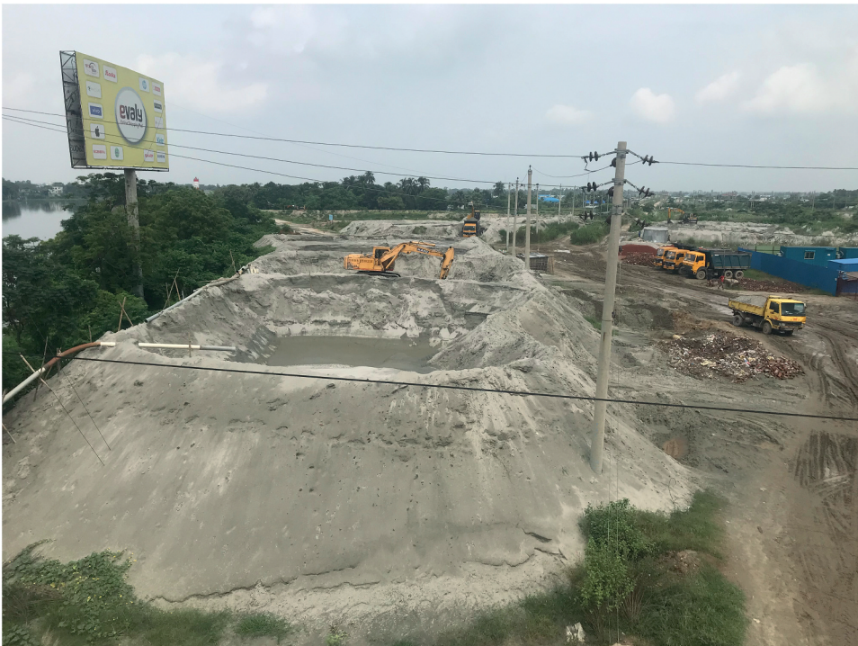
FIGURE 3 Sediment pumping on the Turag River in East Dhaka, October 2019. Photograph by the author.
