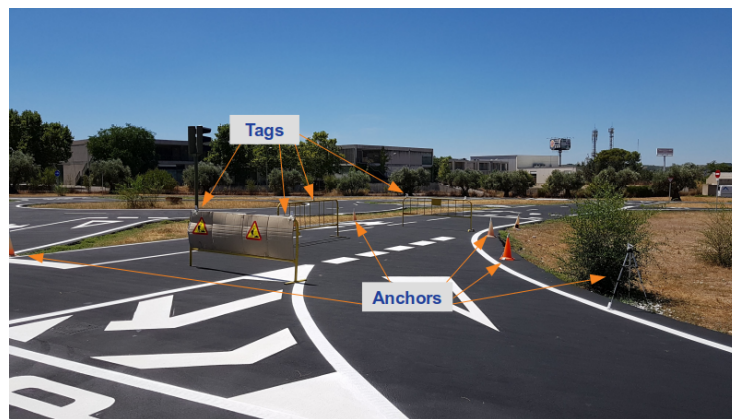
Figure 7. Scenario 1: Roadworks area and UWB sensor.
