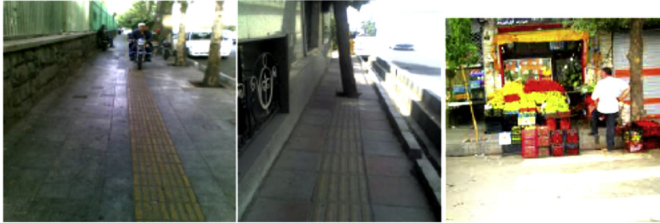
Fig. 1. Examples of obstacles that may cause accident for visually impaired people such as motorbike on the tactile surface indicator (left), a tree at tactile surface indicator and uncovered canal (middle), the whole area of the sidewalk is occupied by shop supplies (right).
