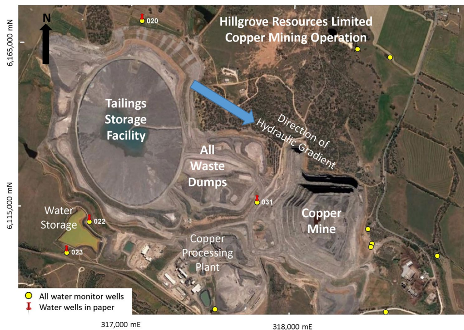
Figure 1. Aerial view of the Hillgrove mine site. Relevant water well sites are labelled. The integrated waste landform, comprising the waste dump and tailings storage facility, is expected on closure to be approximately 75 m above original surface. As of 2014 the foot print of the waste rock dump was approximately 70Ha, with the total footprint of the integrated waste landform being 132Ha. At this time the waste rock was assessed to contain 45.5 Mt NAF (non-acid forming) material and 48.9 Mt PAF (potentially acid forming) material. Image ©2018 Google courtesy of GoogleEarth. Image is dated 15 October 2017. Google Earth has given a general permission for its use in this manner ( https://www.google.com/permissions/geoguidelines/ ). The figure was created using MapInfo Pro software, version 15.0 Build 18, https://www.pitneybowes.com/ie/location-intelligence/geographic-information-system/mapinfo-pro.html .
