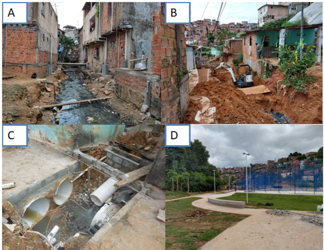
Figure 2. (A,B) An open sewer between households in the study area, (C,D) The study area undergoing environmental modification i.e. channeling of the drainage into a major junction, and the construction of community square, roadway and sidewalk. The figure photographed by Fabio Neves Souza, Institute of Biology, Federal University of Bahia, Brazil.
