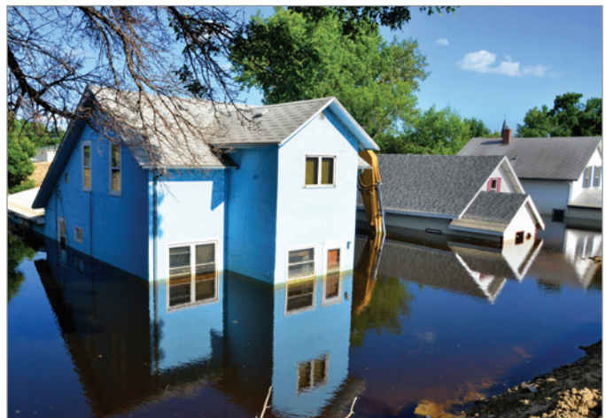
Figure 2. Minot, ND, July 3, 2011. Flood damage in Minot, ND. FEMA is supporting the emergency management team in providing disaster assistance to those affected by the flooding. Photo by: David Valdez/FEMA.
