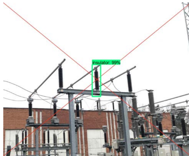
Figure 14. The final output image of the proposed discharge detection system, showing the suspicious element in the center of the image. Deep learning methods are used to determine the origin of the object.
