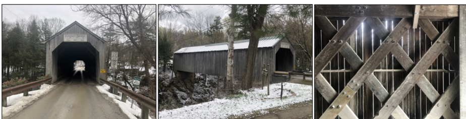
Figure 1. The Kingsley Covered Bridge left and middle images show the historic lattice-truss structure. Right image shows the vertical gaps as seen from the interior of the bridge. Note: While standing still, by default the wall serves as the depth of fixation rendering any potentially visible form-features of the outdoor scene out of focus and nearly invisible. With great effort, I could shift to a distant depth of fixation and experience seemingly random bits and pieces of colour and texture within the gaps.
