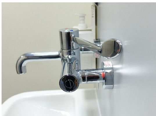
Figure 1. (a) Incorrect set-up of elbow-operated lever which is flush with the inspection panel behind making it difficult/impossible to operate with an elbow. (b) Correct set-up requires an angle of 15° in front of the main body of the outlet linking the hot and cold supply.
