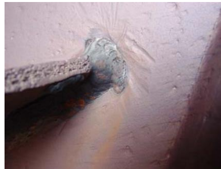
Figure 23. Photo of C fan after repair welding.
