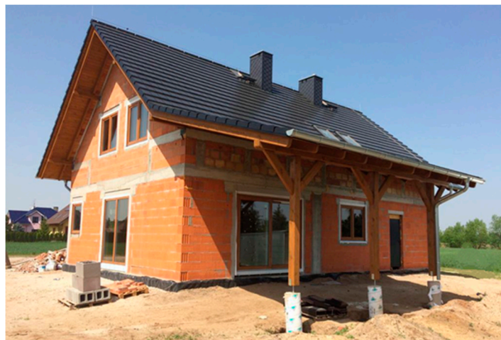
Figure 5. The analyzed building constructed with traditional materials.
