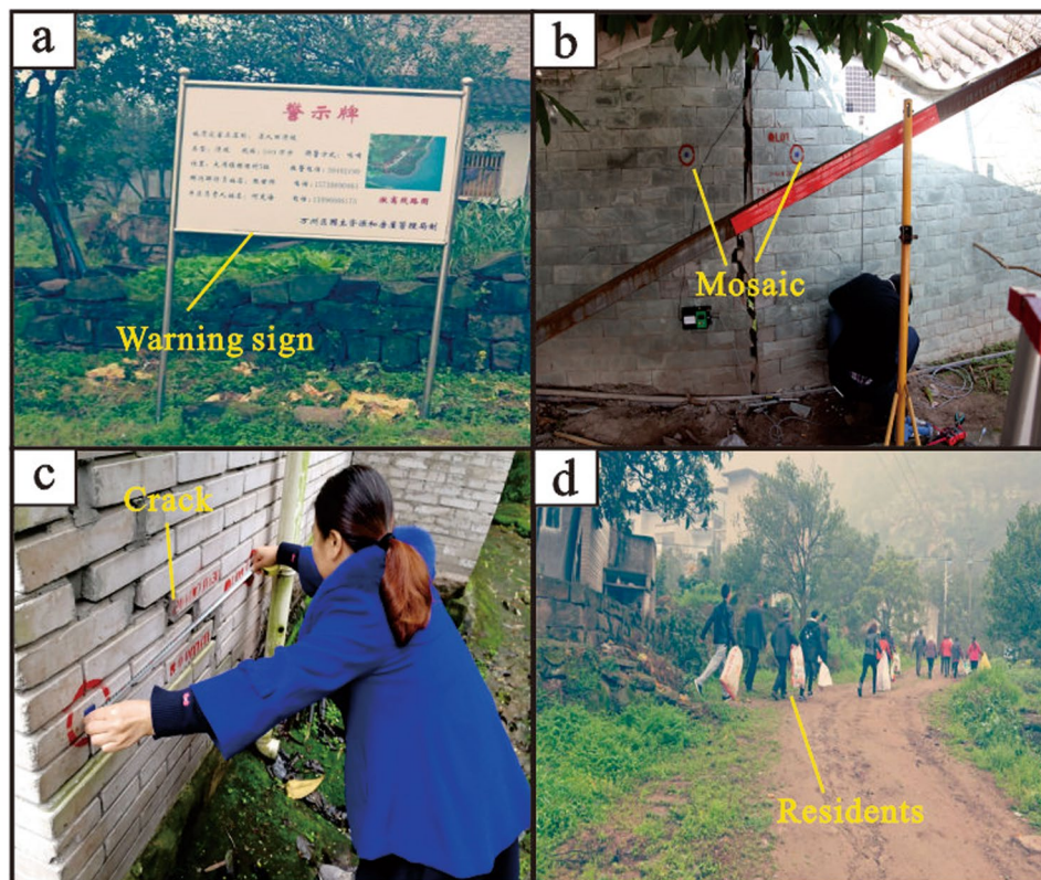
Figure 7. The CBDRR system measures taken in landslides: (a) The warning sign marking the basic information of the landslide. (b) The building crack monitoring using mosaic. (c) The crack monitoring performed by resident. (d) The emergency drilling.
