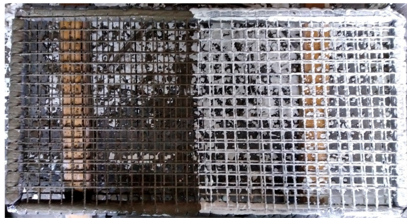
Figure 7. Preparation of reinforcement mesh: (a) Method of carbon mesh preparation (unit: mm); (b) Mesh from carbon roving saturated with cement suspension—surface application by roller (from left): CEM 42.5 R, CEM 52.5 R.
