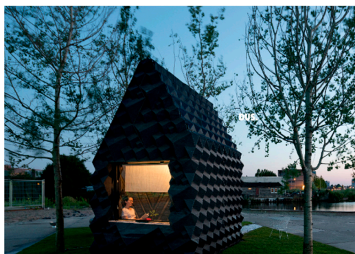
Figure 19. The first 3D-printed house by DusArchitects [201]. Figure reproduced with permissions.
