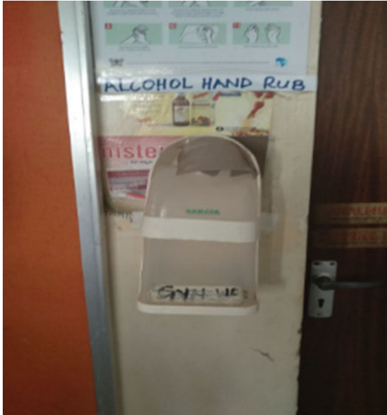
Fig. 4.2 Empty and damaged hand gel dispenser next to Ugandan guidelines on handwashing
