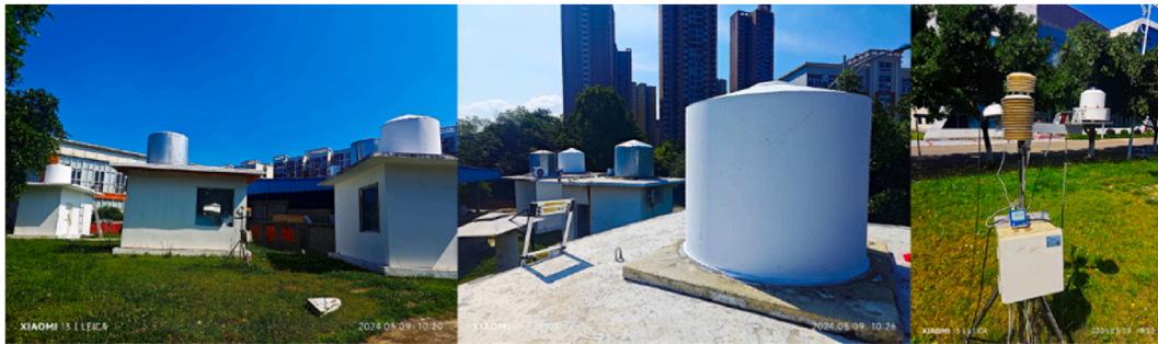
Fig. 1. Photographs of galvanised model silos with different outer thermal layers on roof tops of model buildings and a weather station near the model buildings
