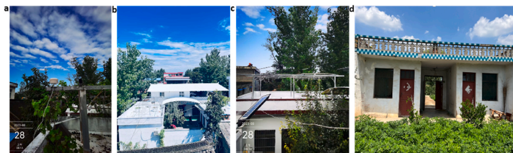
Fig. 2. Photographs of (a) the thermometer screen, (b) panorama and front (c) views of a SSC-HE-coated and (d) a white control brick bungalows.
