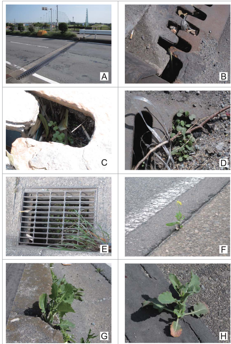
FIGURE 4. Typical habitats of oilseed rape plants in road structures and on the roadside along Route 23. (A) A joining section of the Kumozu-ohashi bridge. The steel frame of the bridge is at the road surface level. (B) A close-up view of a joining section of the Kumozu-ohashi bridge with accumulated mud and sand. (C) Oilseed rape seedlings growing in the mud accumulated at the bottom of the joint. (D) Seedlings and juvenile plants growing in the mud accumulated in a drain. (E) Densely populated square pond connected to the drain. (F) An adult plant flowering in a chink between asphalt pavement and curbstones. (G) An adult plant just before flowering in a crack in a curbstone. (H) An adult plant just before flowering in a crack in a rubber seal that coated a chink between curbstones to prevent weed growth.
