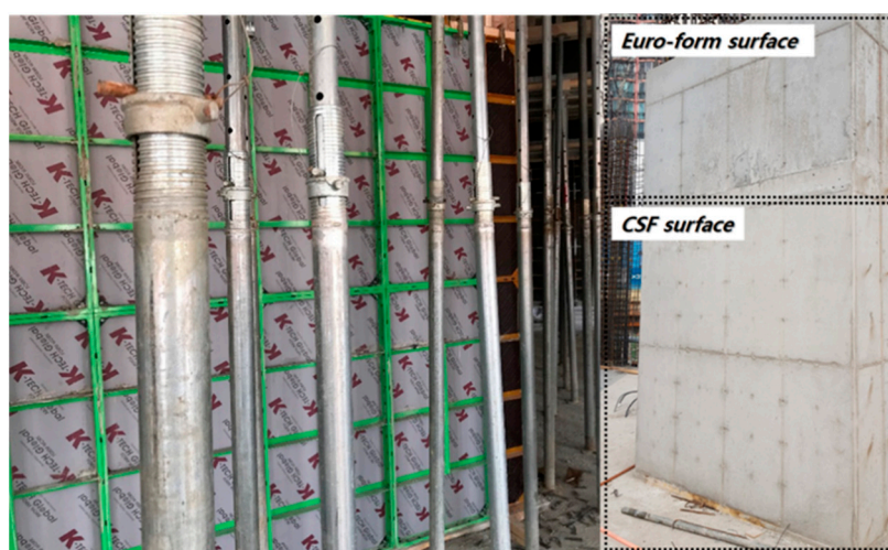
Figure 12. Concrete surface quality comparison between the CSF and the Euro form.
