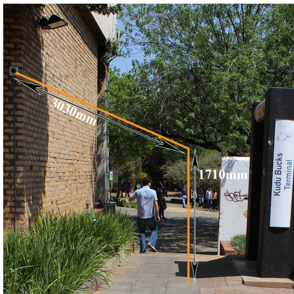
Figure 4. Demonstration of estimated objective to face distance at site A. Vertical distance indicates the mean height of a South African male (1710 mm) and the oblique distance indicates the calculated approximate camera to face distance at Site A (3030 mm).
