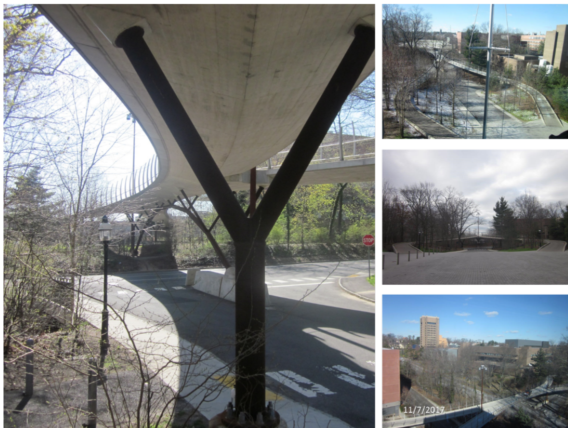
Figure 4. Photographs illustrating complex 3D geometry of Streicker Bridge [37].
