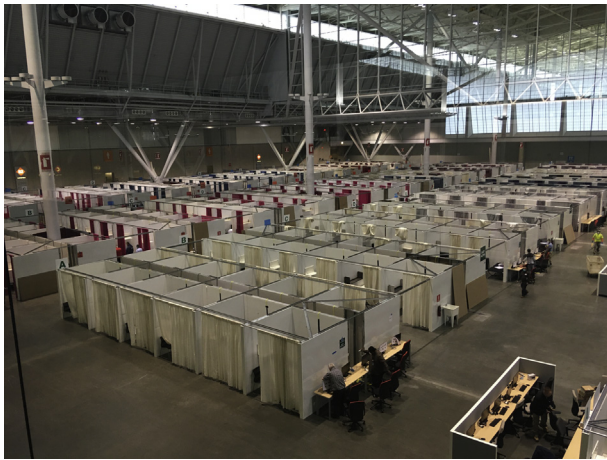
Fig. 1. Photograph of the field hospital in the final stages of construction. A downloadable PDF of this form is available at www.sciencedirect.com . Boston Hope
