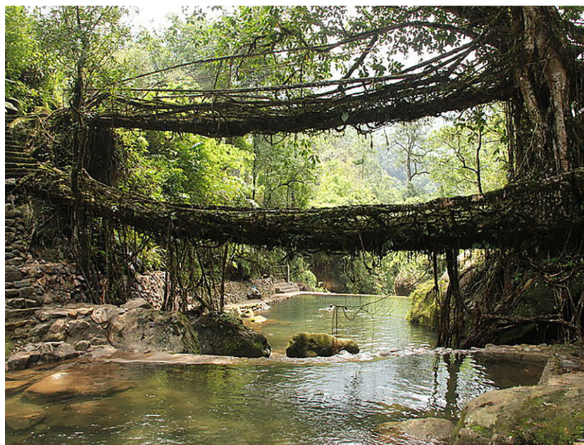
Figure 5. One of the Living Root Bridges constructed by the manual rearrangement of root growth over long periods of time [209]; image used with license. (Image retrieved from Wikimedia Commons, attributed to Arshiya Urveeja Bose. Used with Creative Commons license CC BY 2.0. Image copyright holder chose and approved the license at upload.) (Online version in colour.)
