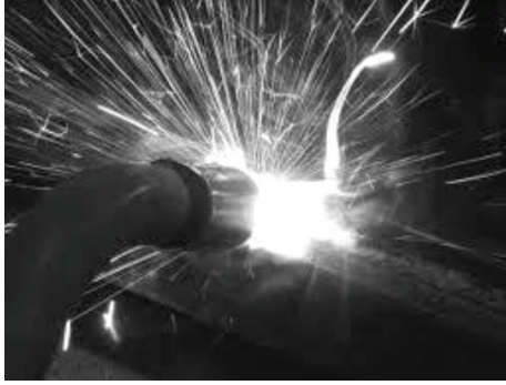
FIGURE 2: Opening for electric arc welding activity.
