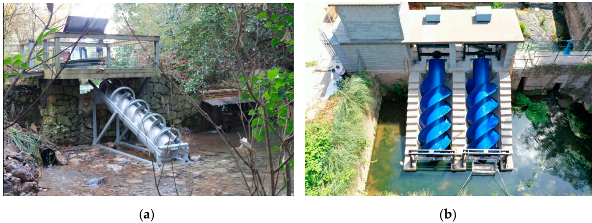
Figure 4. AST experimental prototypes. (a) Atlantic Botanic Garden of Gijón (Spain); (b) Barreda hydroelectric plant in Torrelavega (Spain).
