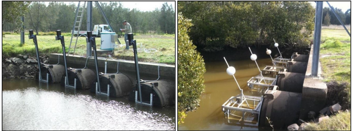
Fig 6. Electronic SmartGates at Stage 1 (left) and buoyancy controlled SwingGates at Stages 2 and 3 (right).
