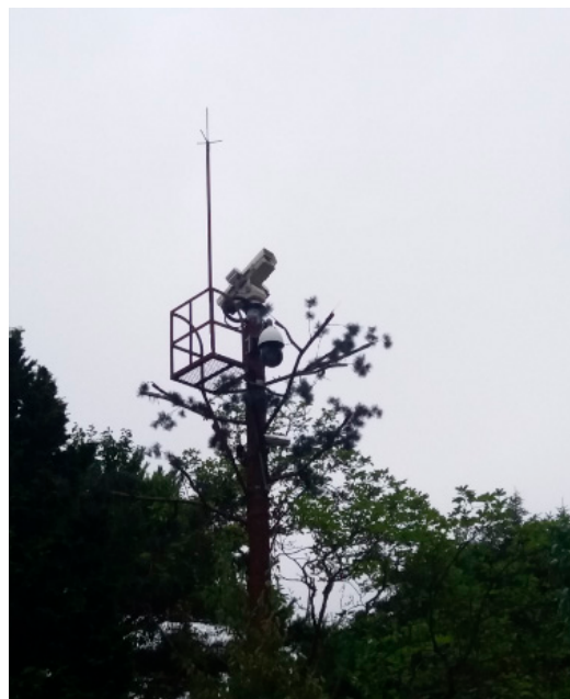
Figure 2. The power-line communication (PLC)-based lightning rod and intelligent closed-circuit television (CCTV) system installed at Beomeosa Temple (Geumjeong Mountain, Republic of Korea (ROK)) for a test bed experiment.
