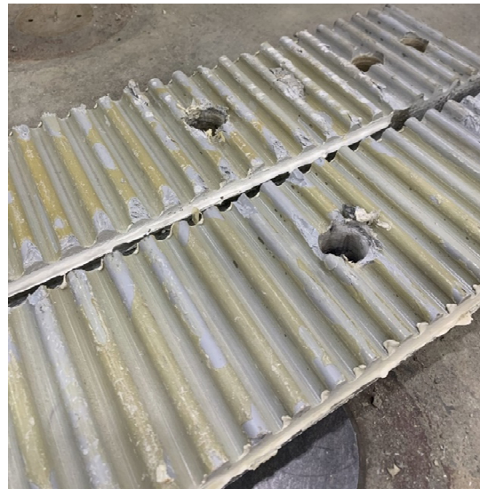
Figure 1. Deformed FRP Girder Top Flanges Used in Shear-Friction Connection.
