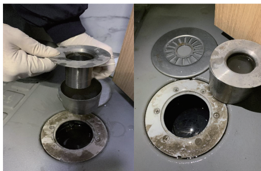
SUPPLEMENTARY FIGURE S5. The figure of the floor drains and removable water trap in a centralized quarantine apartment in Beijing.
