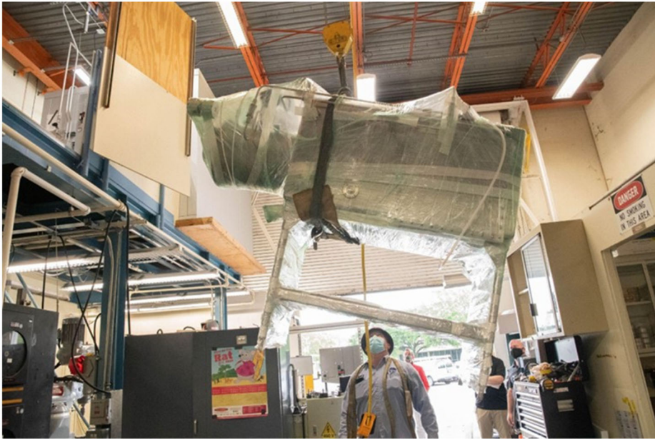
Fig. 19 Glovebox being lifted to the EIL mezzanine; sample processing freezer is visible on the mezzanine level at the upper left
