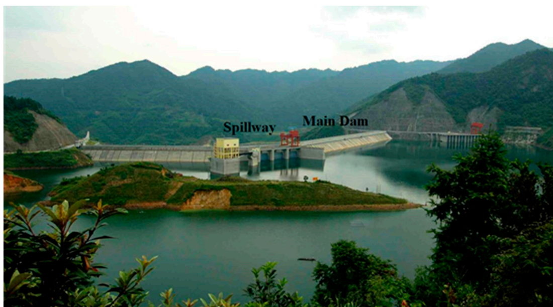
Figure 3. Upstream of hydropower station dam.
