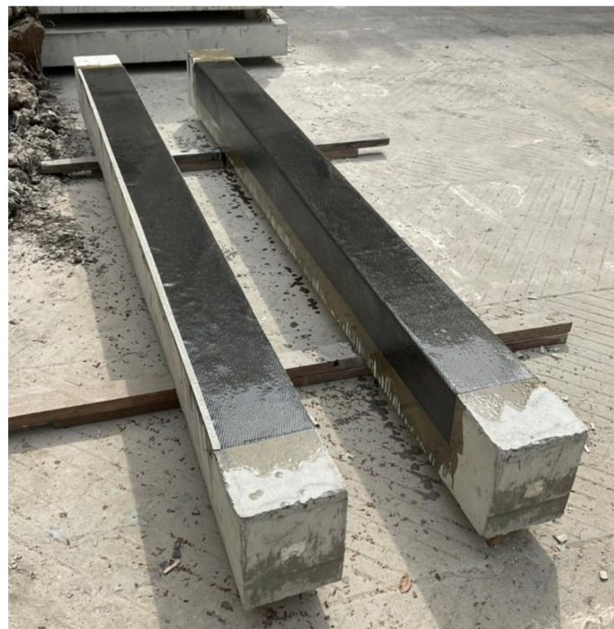
Figure 3. Application of CFRP sheet on bottom of beams (left) tension side only (right) u-shape sheet.
