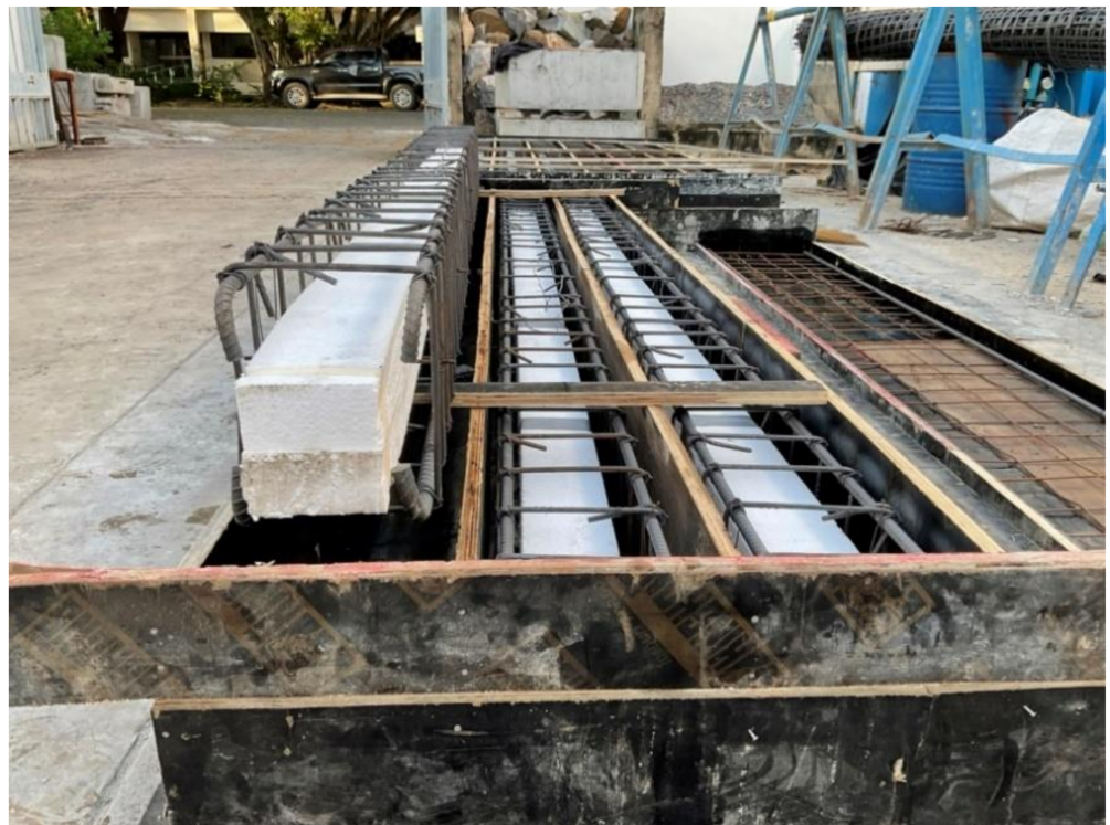
Figure 4. Installation of foam in steel bars.
