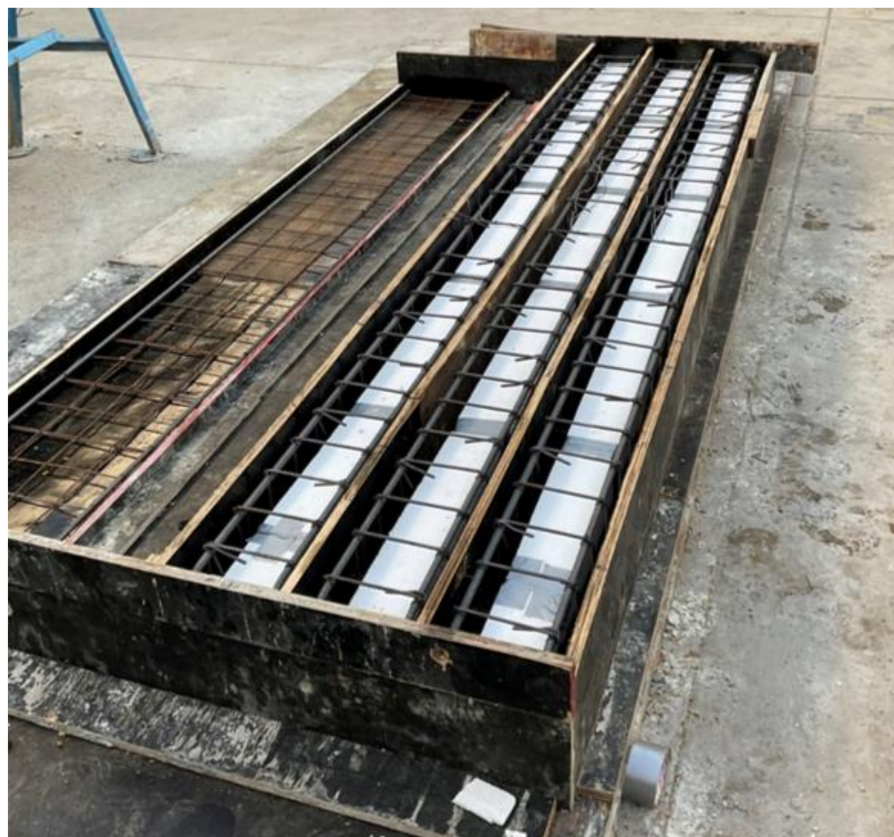
Figure 5. Installation of steel bars in formwork.
