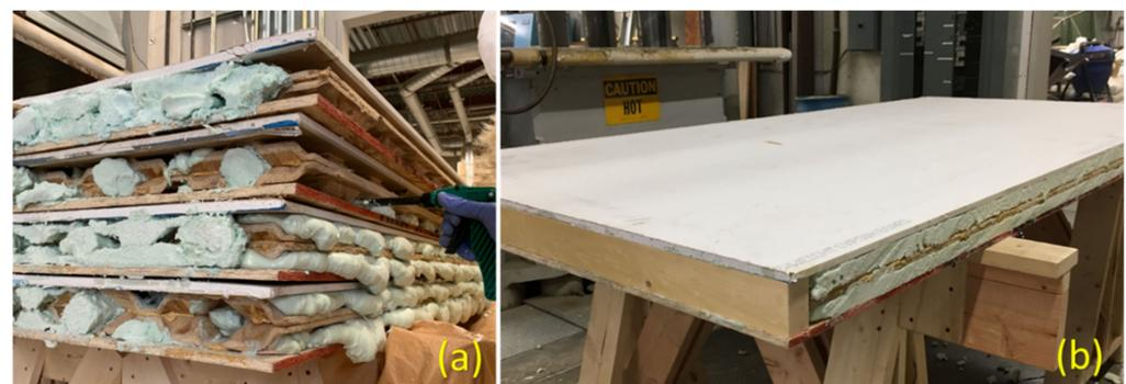
**Figure 4.** (a) Filling two-layered core sandwich panels with spray foam (b) trimmed foam and wall prepared to use.
