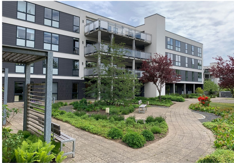
Fig. 5 View from the pergola of the most of 'Section 2'
