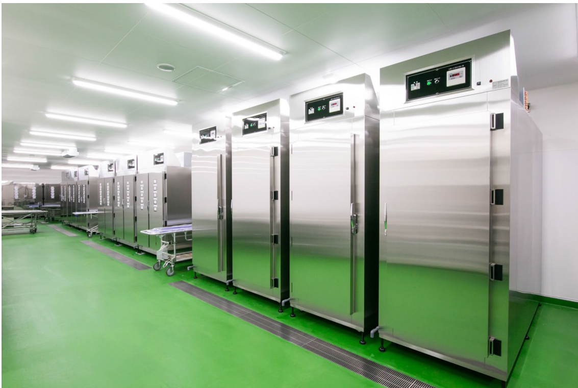
Fig. 9 Mortuary. The mortuary has ten mortuary cabinets (100 bodies), six refrigerators (60 bodies), and six freezers (30 bodies)
