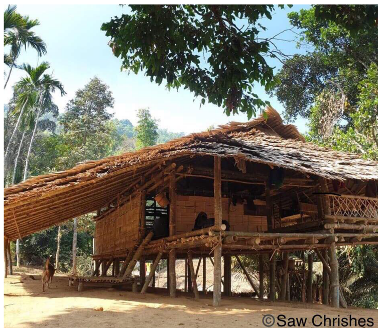
Fig. 4 Typical bamboo housing with a leaf roof and bamboo walls and floor
