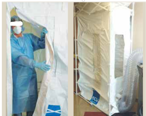
Figure 5. Temporary negative pressure isolation: although not as suitable as permanent ventilation solutions, a portable anteroom may be installed and connected to portable air ducts. Reproduced from public reference (7). (Color version of figure is available online.)
