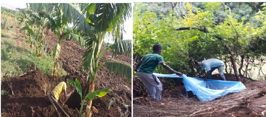
Fig. 2. Construction of pit shelter for outdoor resting mosquito collection under the shade (left) and collecting mosquitoes by closing the mouth of pit shelters by white sheet (right).
