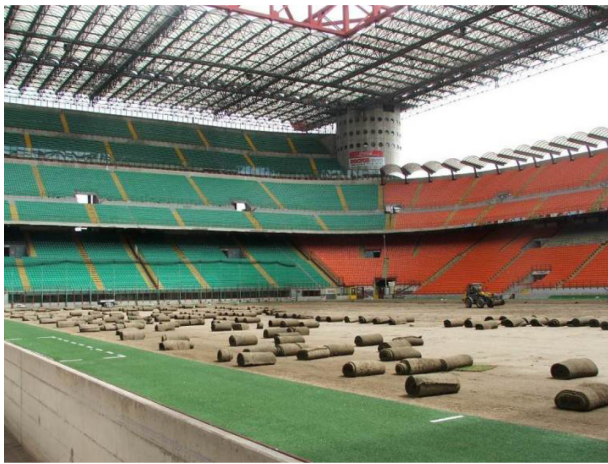
Figure 12 Portable natural grass being laid in rolls at the San Siro, Milan.
