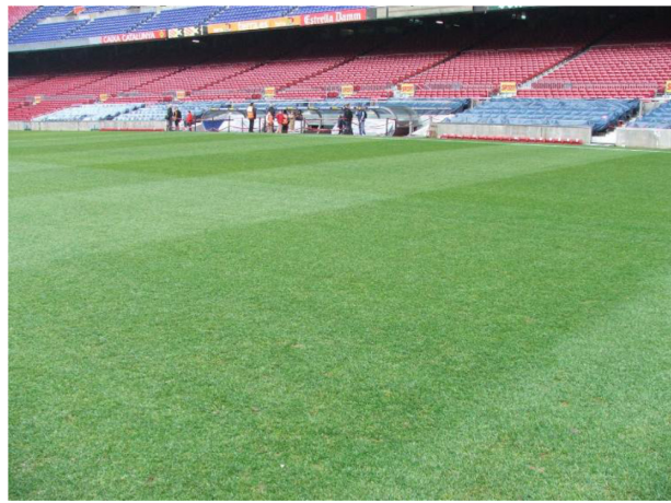
Figure 14 Squares in situ with no joins visible surface.
