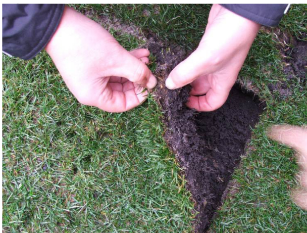
Figure 13 Portable squares being laid at the Nou Camp, Barcelona.
