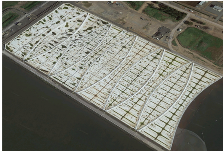
Figure 1. Illustration of HDPE floating cover in the WTP.
