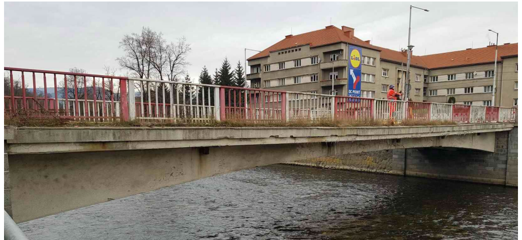
Figure 3. View of the bridge.
