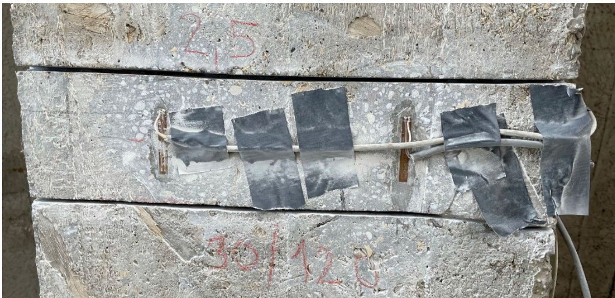
Figure 10. View on performed saw-cuts and installed strain gauges.
