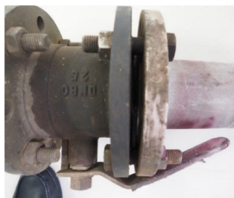
Figure 11. Connection condition between the ball valve and the flange.
