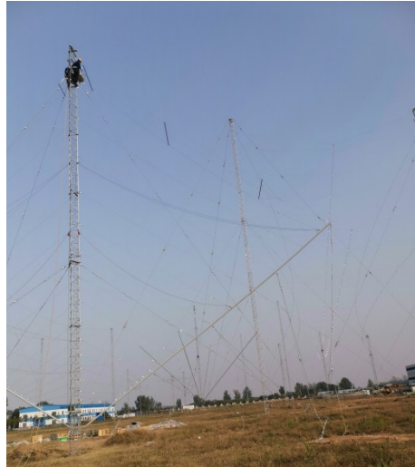
Figure 10. Fabricated miniaturized transmitting LPDA.
