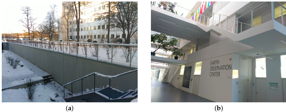
Figure 11. (a) shows the three outdoor stairs of the building and (b) shows the two indoor stairs.
