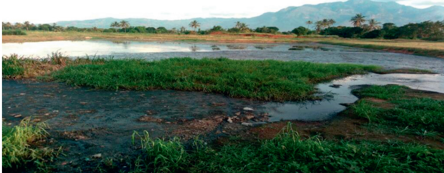
FIGURE 5: Anaerobic pond of Morogoro WSPs showing accumulated sludge (photos taken by first author during sample collection).
