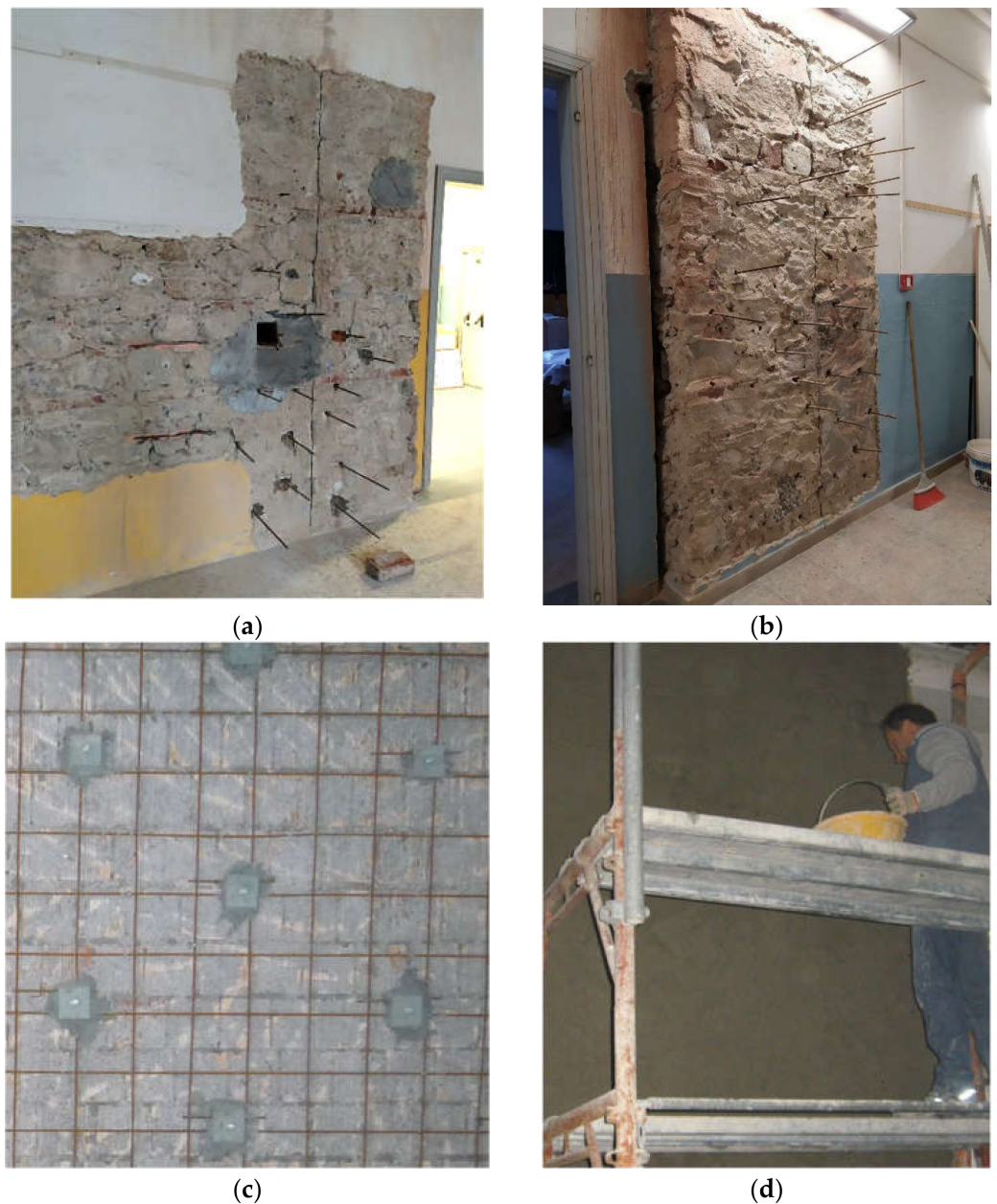
Figure 6. Strengthened technique adopted to restore the tested walls: repair of cut and cavity (a), insertion of threaded or reinforcing steel bars (b), application of the reinforcing steel mesh (c), and final grouting of the concrete layer (d).
