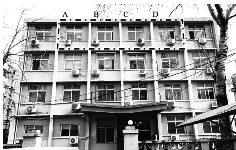
Figure 10. Field study rooms (room A: SG, room B: SG + F, room C: DG, and room D: DG + F).
