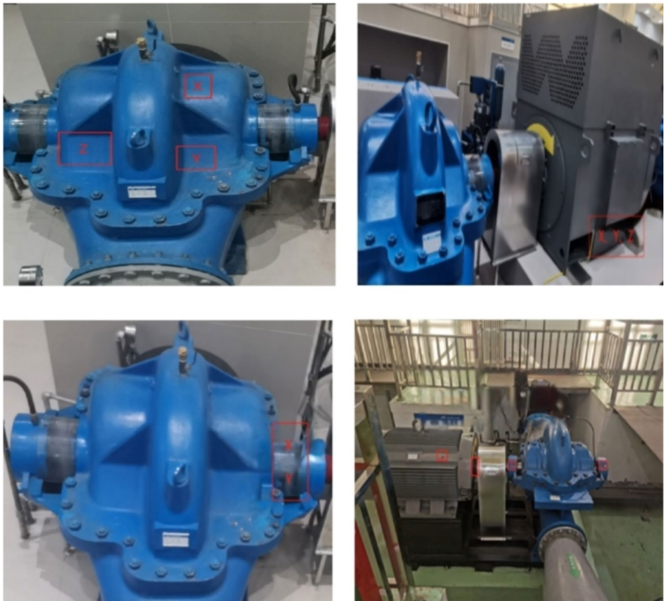
Fig. 6. Schematic diagram of PSUs components and sensor array on site.
