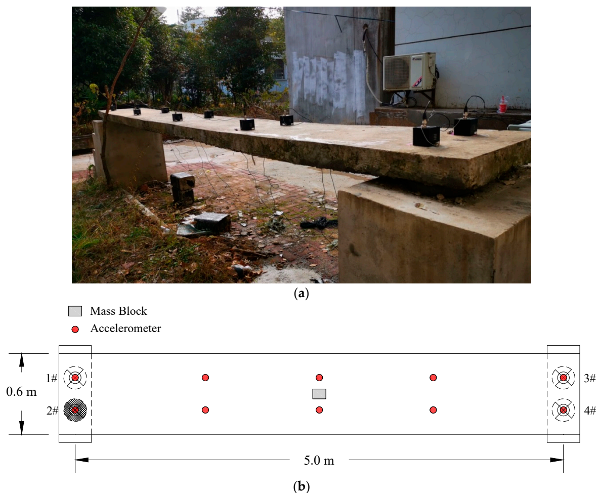
Figure 10. The simply supported reinforced concrete plate: (a) view of modal test; (b) layout of sensors and mass block.
